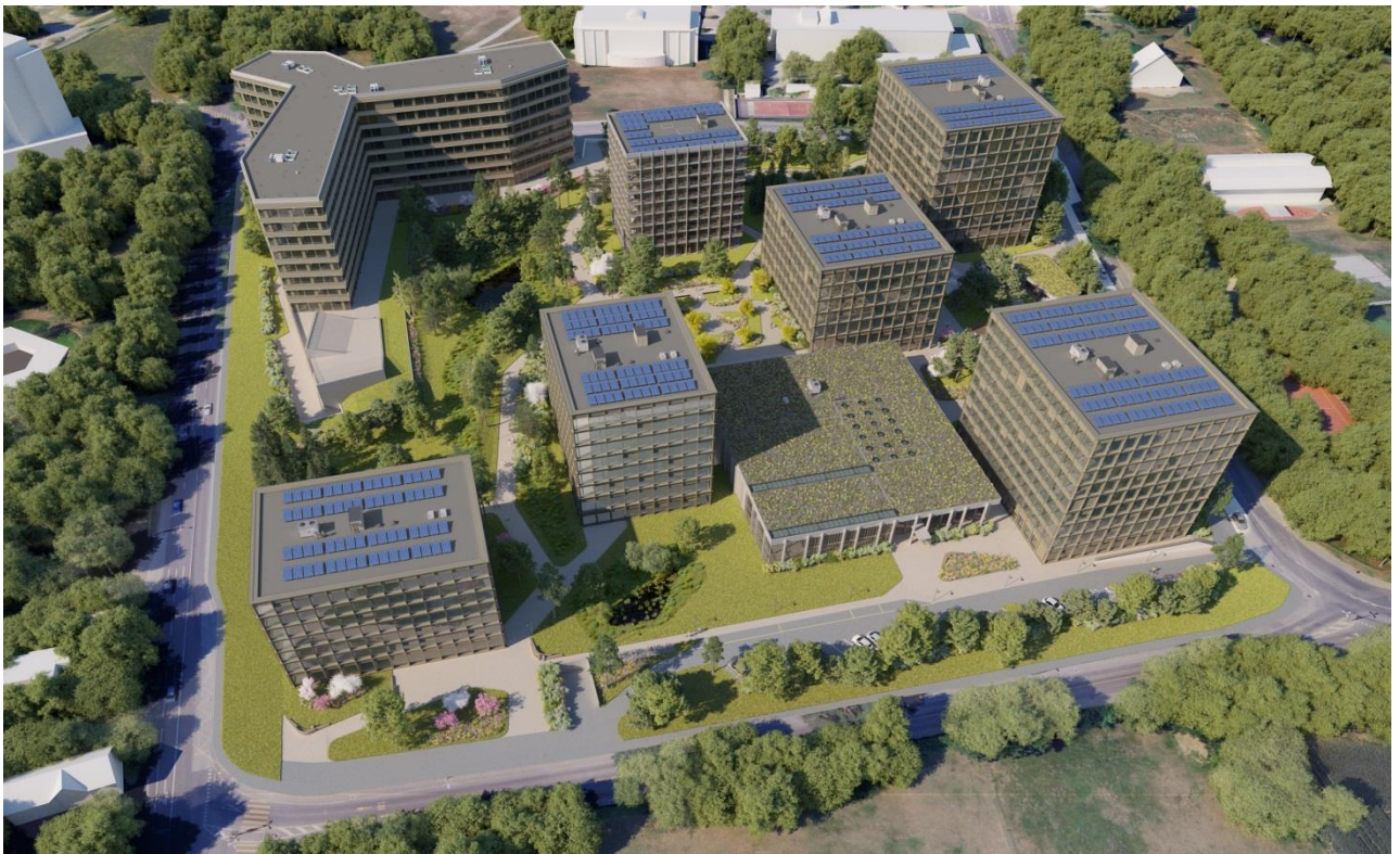
The Green Village project includes administrative buildings, a hotel and a residential building. Located in the heart of Geneva's international district, it is set in a landscaped park. (Image: Implenia)
