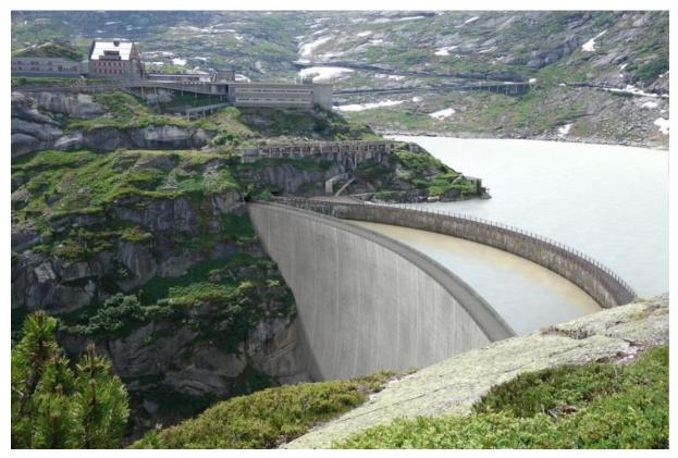
The new double-curvature arch dam is to be built directly in front of the old dam wall. The old dam will remain in place and will be filled in on both sides. (Image: KWO / David Ormerod)
