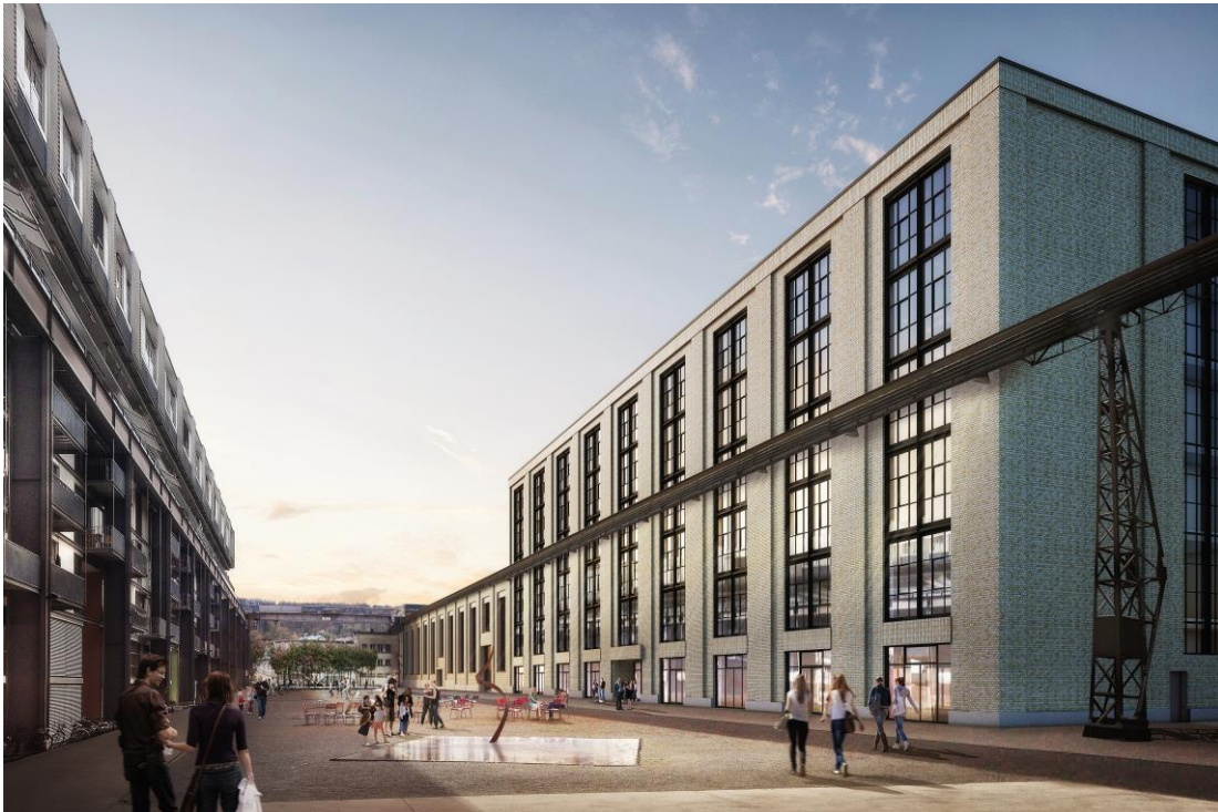
The construction of Haus Adeline-Favre by Implen is progressing right on schedule. It will be Switzerland's largest training centre for occupational therapy, physiotherapy, midwifery and nursing.
