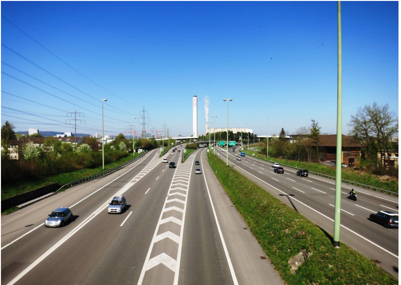
A consortium led by Implenia is upgrading the A1 between Zurich-Ost and Effretikon. (Photo: Implenia)
