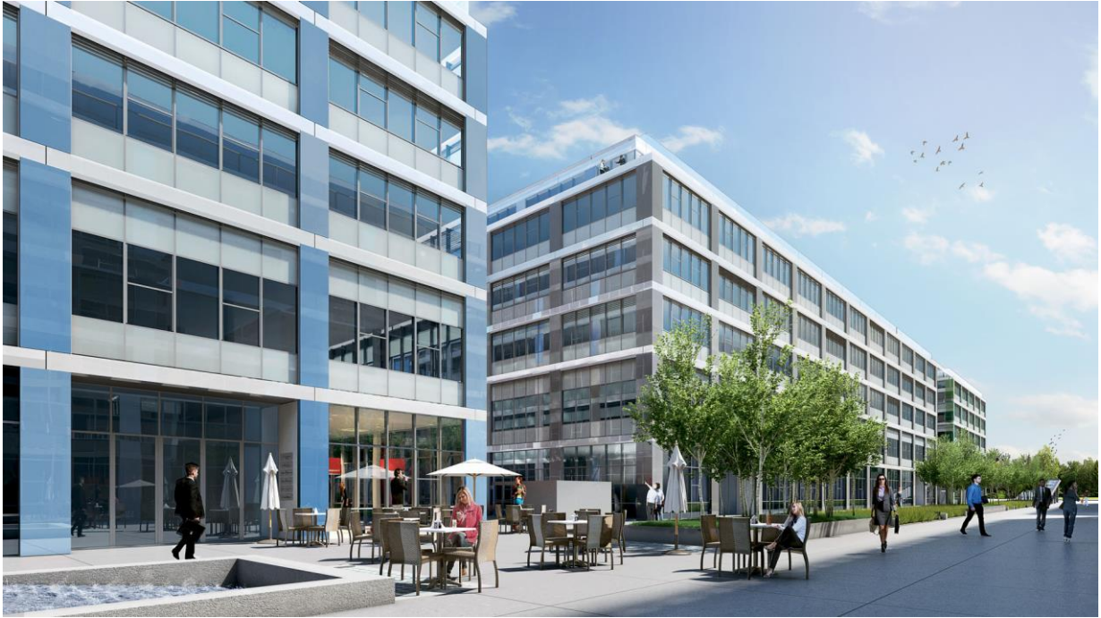
Five buildings providing commercial and office space are being created in Geneva. Real estate company SPS has commissioned Implenla to execute the "Espace Tourbillon" project. (Picture: SPS)
