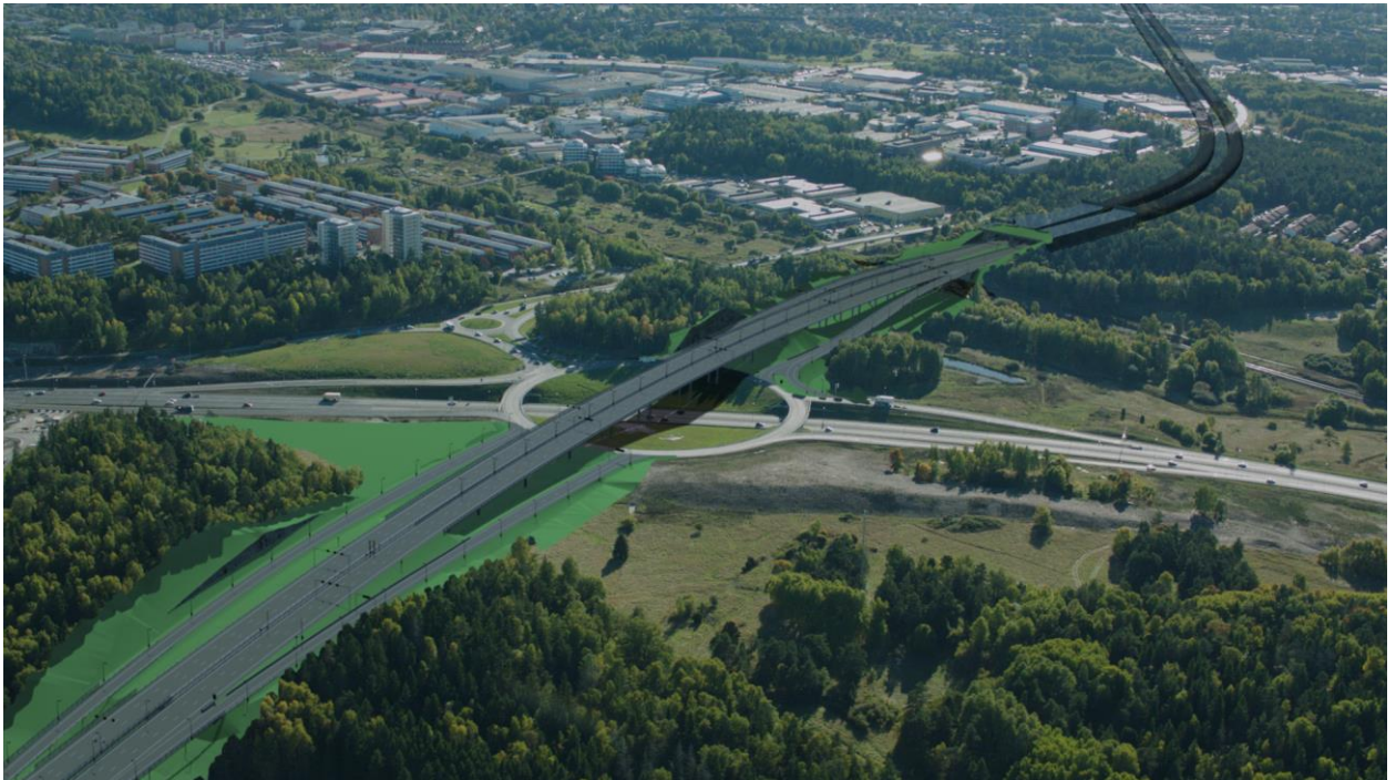
Implenia, working within a consortium, is building the Södra Hjulsta motorway junction in Stockholm on behalf of the Swedish Transport Administration. (visualisation: Trafikverket)
