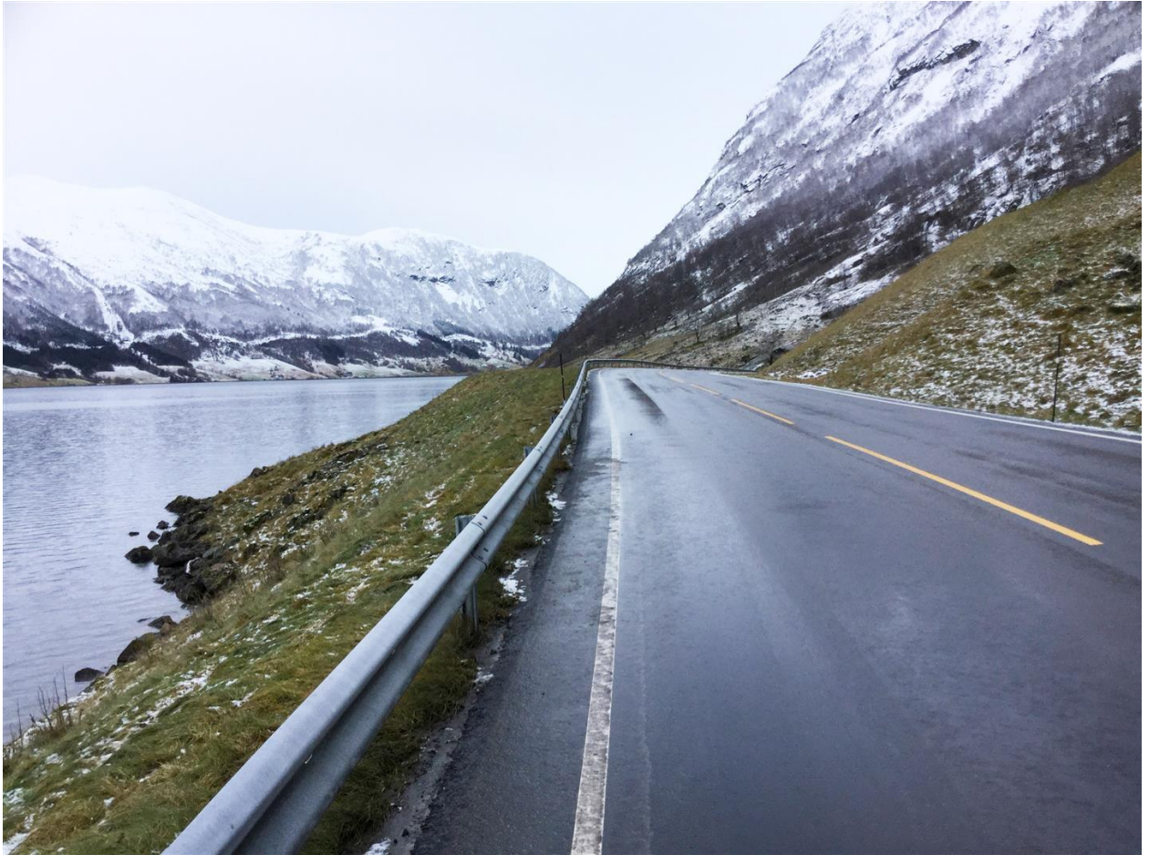
Implenia has been asked to rebuild another section of the E39 road link between Bergen and Trondheim. (Picture: Implenia)
