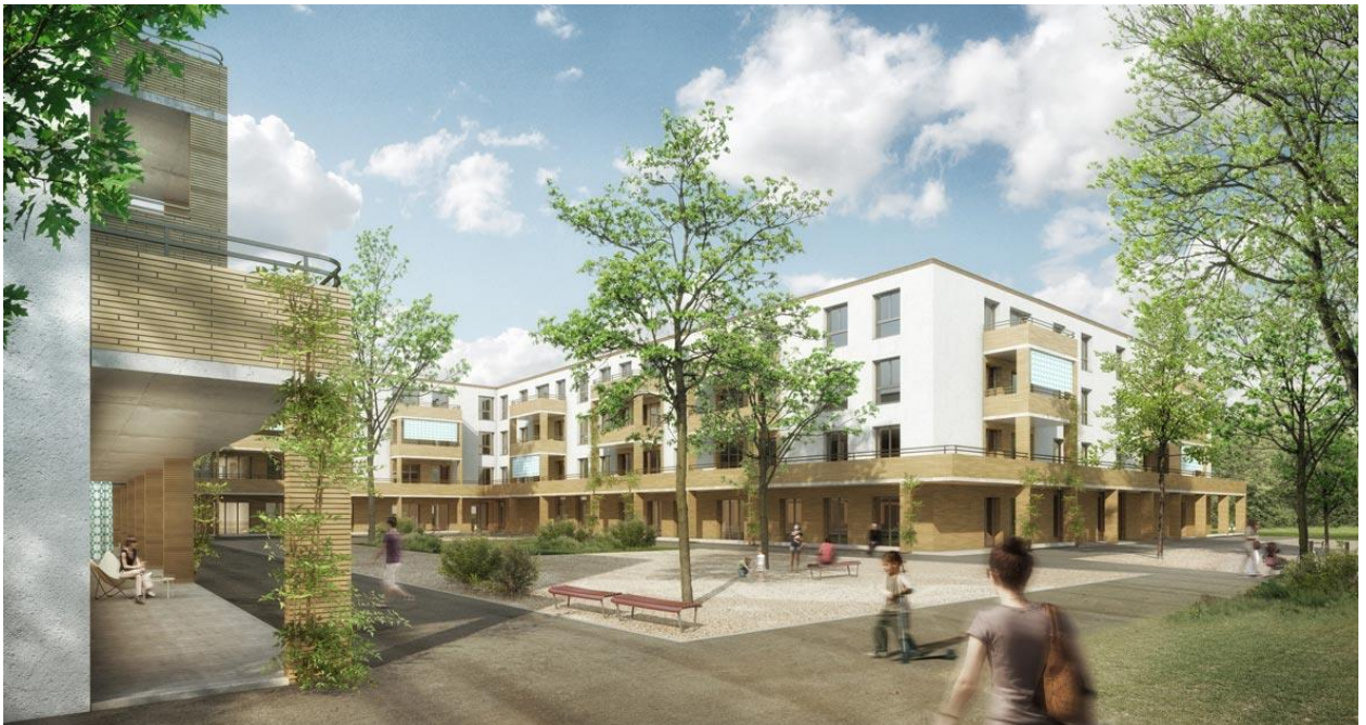
The six four- and seven-storey buildings will ensure future residents have more living space per square metre of land. (Image: pool Architekten, Zurich)
