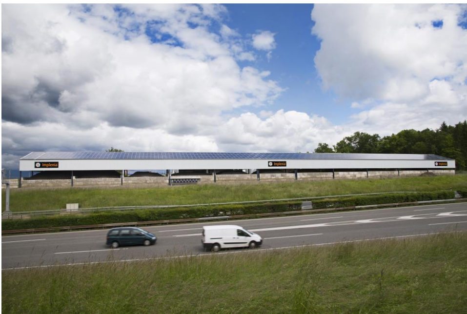
The 2,500 m 2 photovoltaic system on the roof of the surfacing works can be seen from the A1 motorway. It produces more than 300,000 kWh of solar energy every year. (Picture: Implenia)
