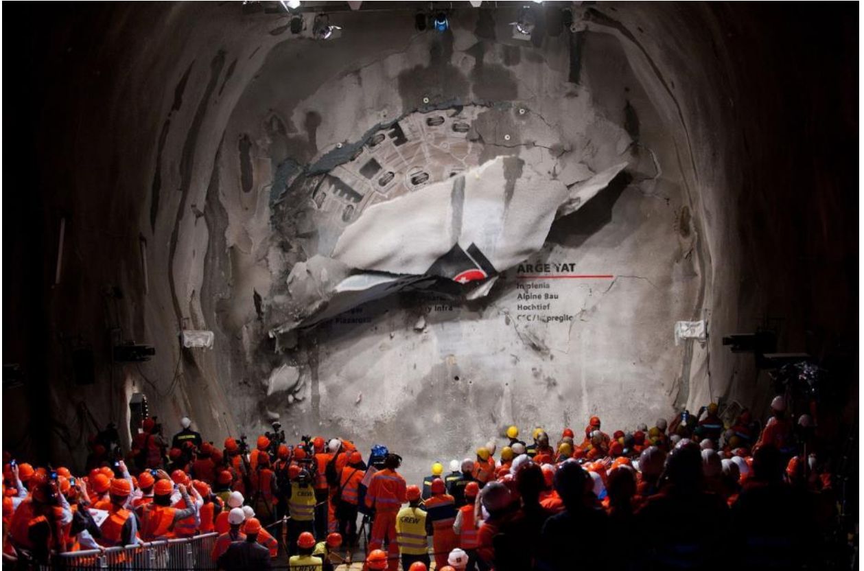
The finished Gotthard base tunnel was officially opened today, almost six years after the tunnel breakthrough in Sedrun on 15 October 2010 (picture). Implenias was heavily involved in three of the five tunnel sections. (Photo: AlpTransit Gotthard AG)
