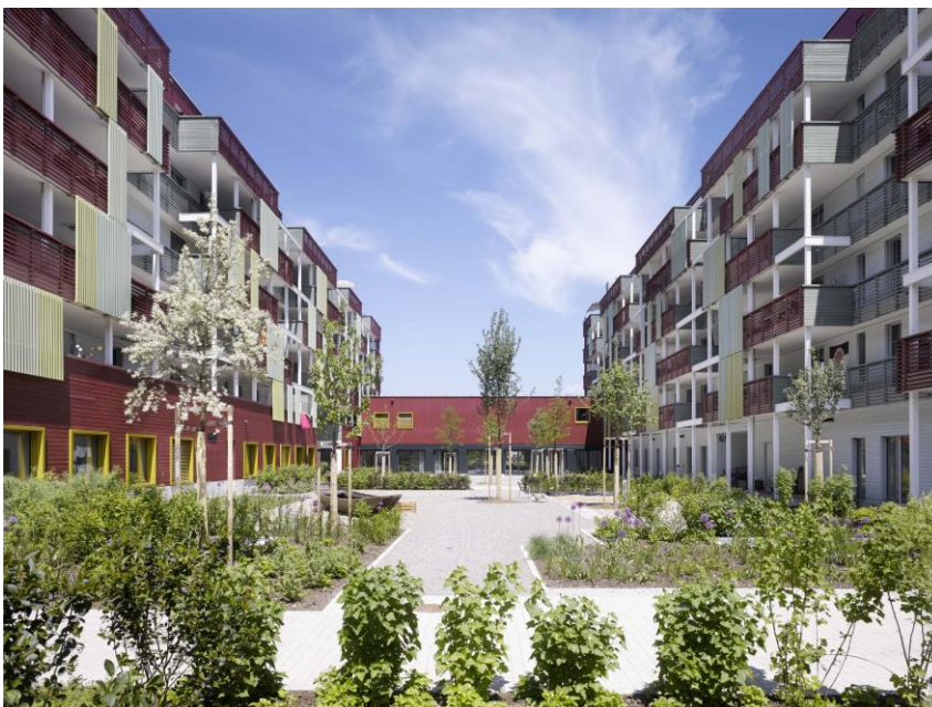
At the Giesserei in Winterthur, everything except the basement floor and the stairwells is made entirely of wood. Implenla Wooden Construction played a major role in the project. (Source: © Hannes Henz, Zurich/Prix Lignum 2015)
