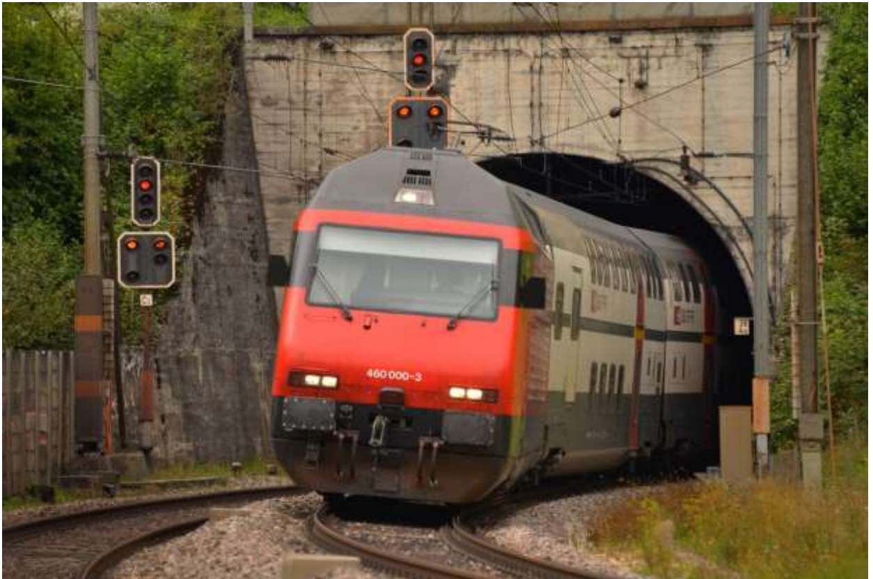
Drilling work on the new Bözberg rail tunnel starts here at the southern portal near Schinznach-Dorf in spring 2016 (picture: Stefan Wullschleger).
