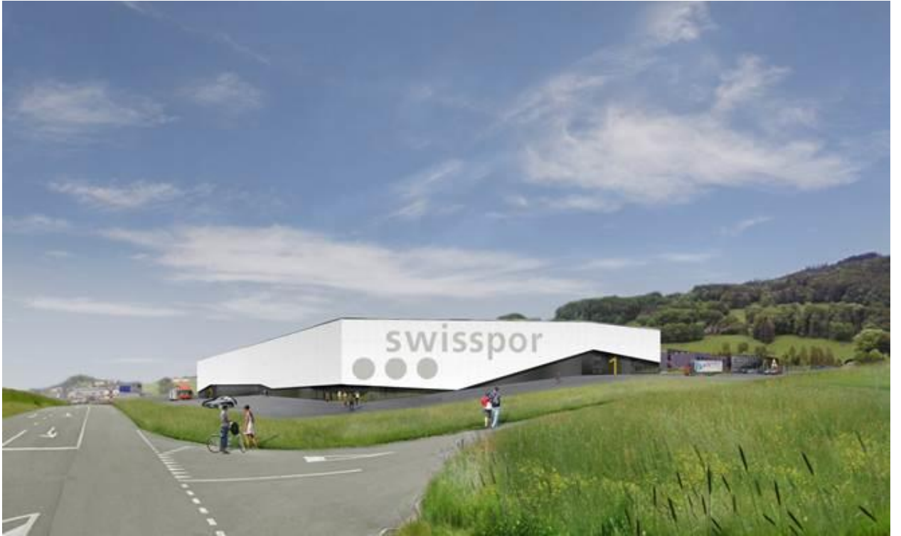
The seemingly random juxtaposition of dark and light surfaces lightens the appearance of the future swisspor production site in Châtel-Saint-Denis.
