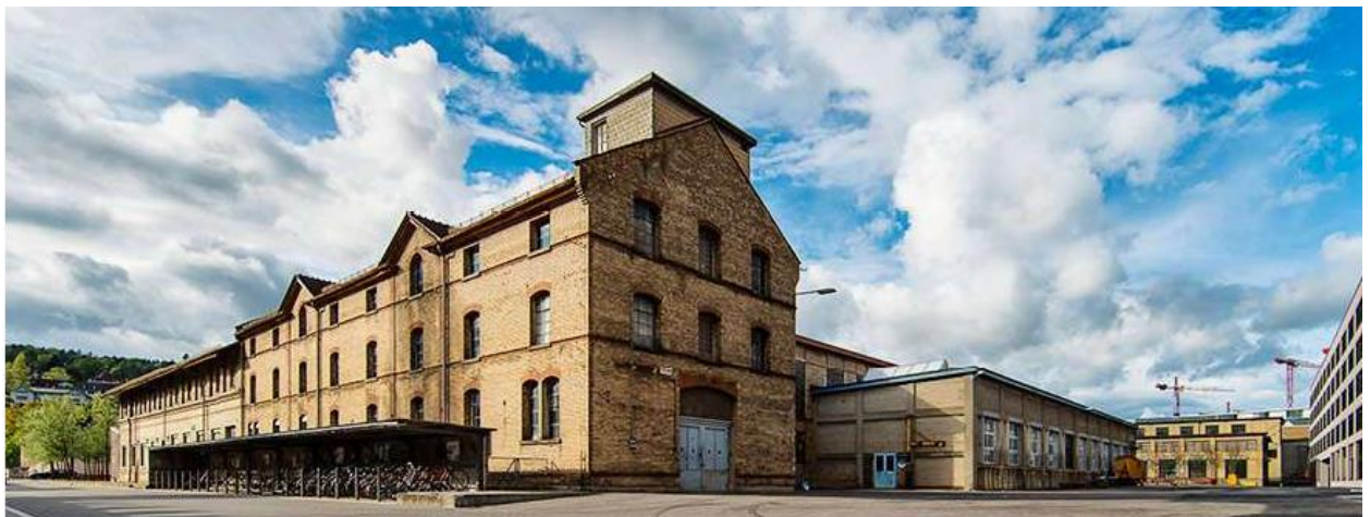
The first 2000-Watt quarter in Winterthur is being built on the Werk1 plot over the next few years.
