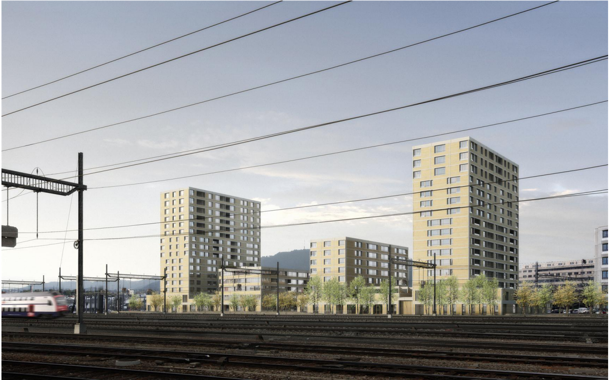
Implenia is carrying out a major project for Swiss Federal Railways in Zurich Altstetten.
