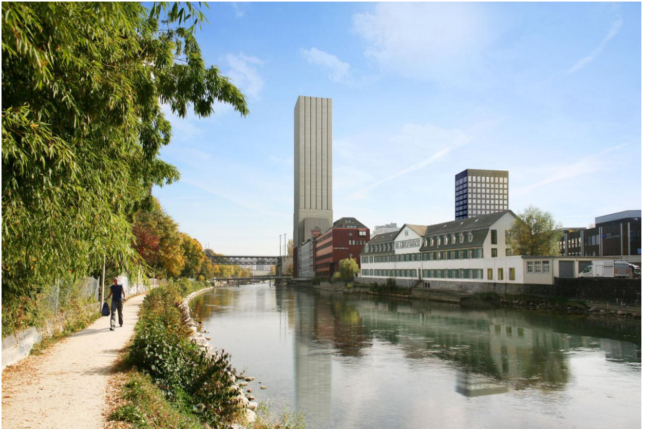
Implenia enlarges the Kornhaus in Zurich from 40 to 118 meters.
