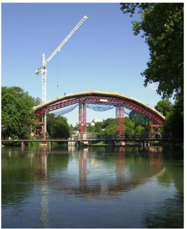
Falseworks are auxiliary structures that are used, for example, for shuttering and concreting when building concrete bridges.
