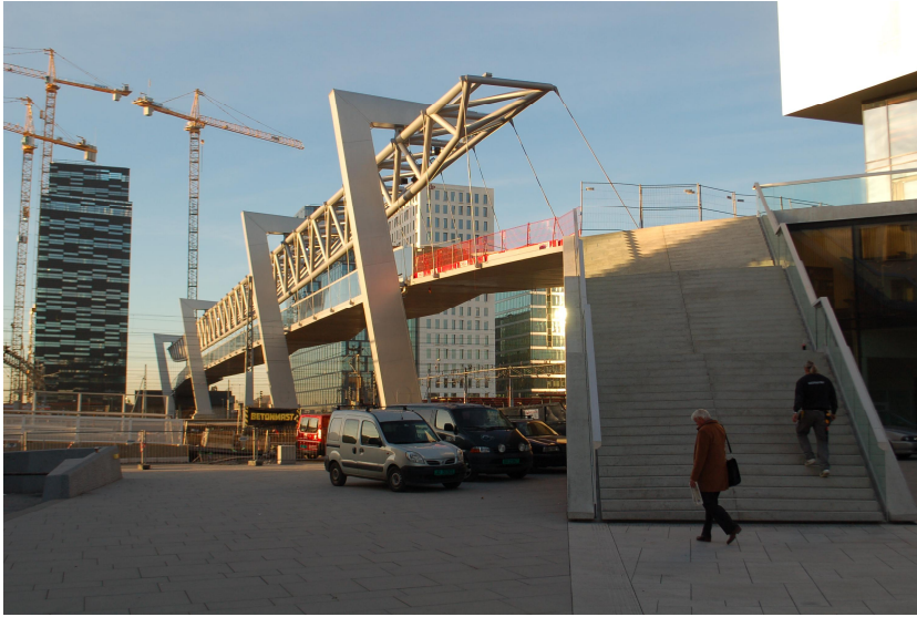
Implenia received the European Bridges Award for the "Acrobats" footbridge in the centre of Oslo.
