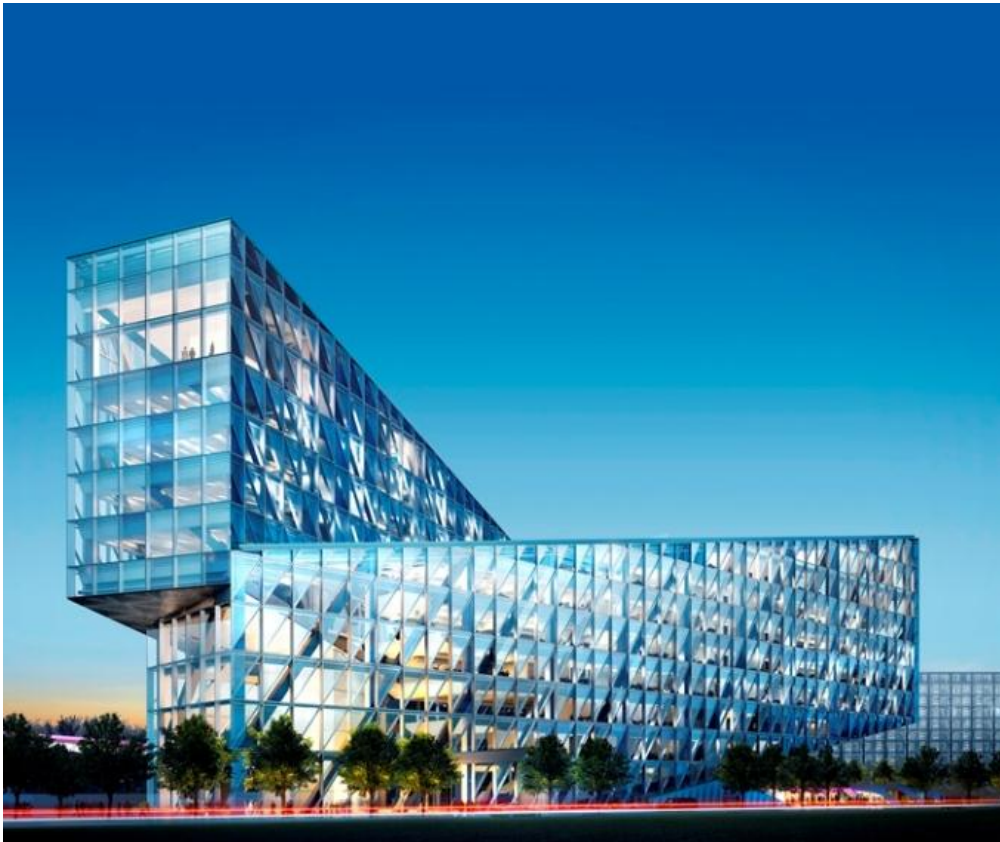
JTI's future international headquarters in the Sécheron area of Geneva. (Copyright : SOM)
