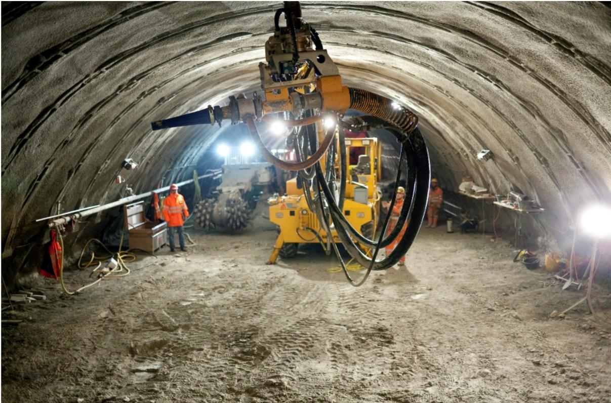
Underground construction of the Lucerne central rail line: the top-down method under pressurised conditions used for the first time in Switzerland had two distinct advantages. Firstly, the groundwater was spared and, secondly, the carcass construction was completed one year earlier than planned.
