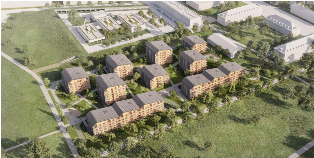
Implenia is building 225 residential units using a timber-hybrid method at the Spinelli development in Mannheim (image: ©design: mvm+starke architekten / visualisation: reinraumimages).
