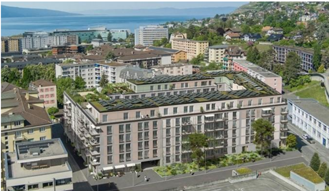
The “Jardins en Ville” project in Vevey, where Implenia is building 182 condominiums as total contractor (image: ©Jardins en Ville).
