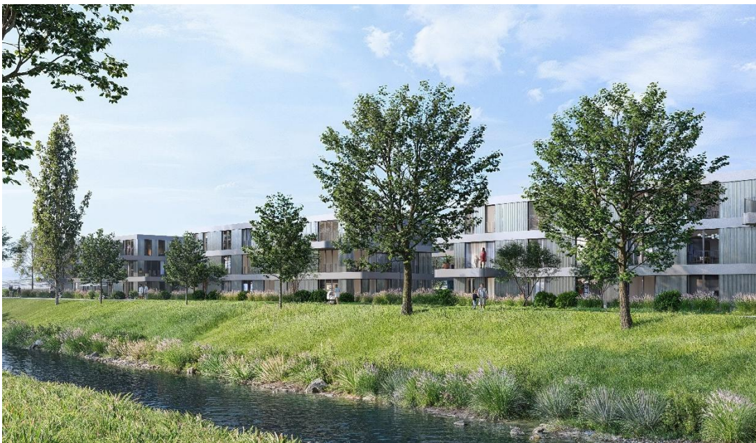
Implenia, as a total contractor is building attractive, sustainable homes in Payerne in French-speaking Switzerland, including rental apartments, condominiums and senior citizens' apartments (image: ©Uzuffy).
