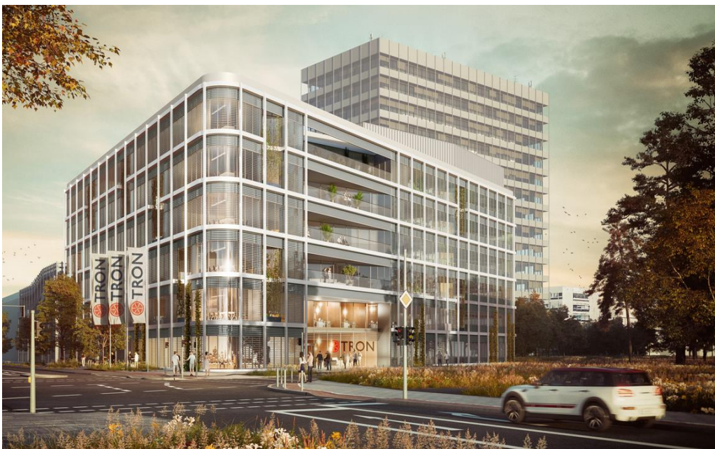
The new TRON research building for cutting-edge medical research in Mainz (image: ©NICKL & PARTNER ARCHITEKTEN AG).
