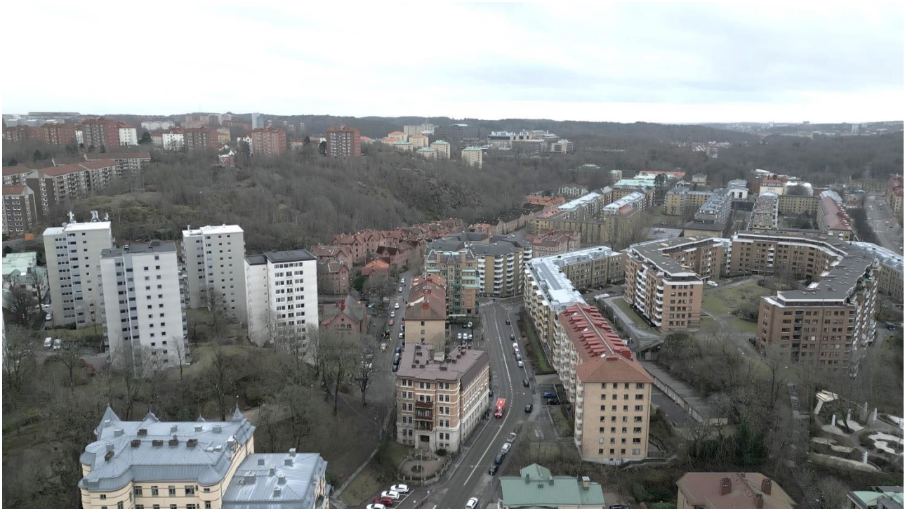
Implenia is building a railway tunnel and the Haga commuter station beneath the Vasastan district of Gothenburg, Sweden's second largest city (image: ©Trafikverket.se).
