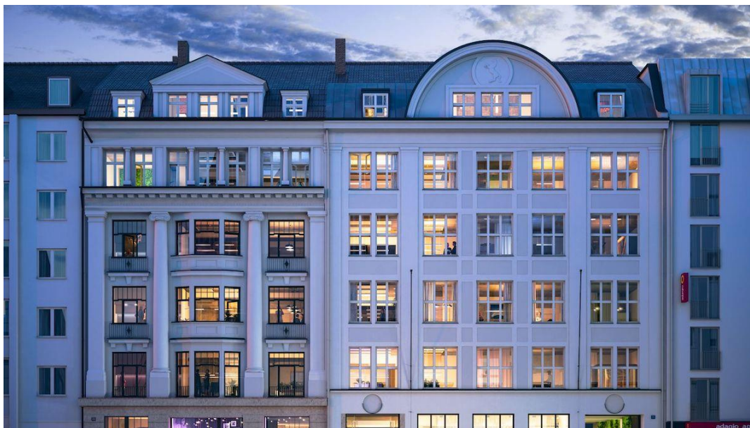
Implenia is renovating two listed properties on Schwantalerstrasse in Munich (image: ©COMM AG).
