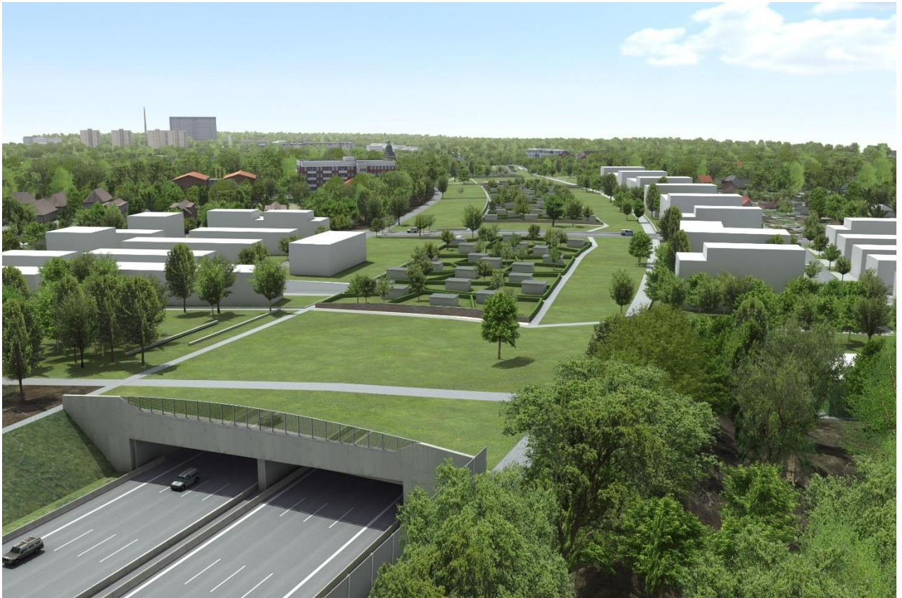
A7 Altona Tunnel in Hamburg: noise protection tunnel covered with allotments, greenery and parks (Image: © DEGES/V-KON.media).
