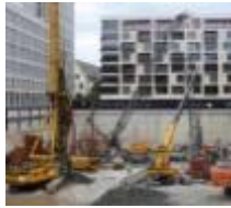
Total construction pits
