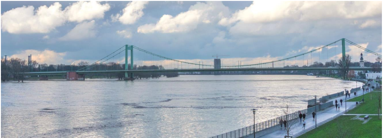
Implenia is renovating the Mülheimer bridge in the north of Cologne from the ground up. (Picture: Björn Krause)
