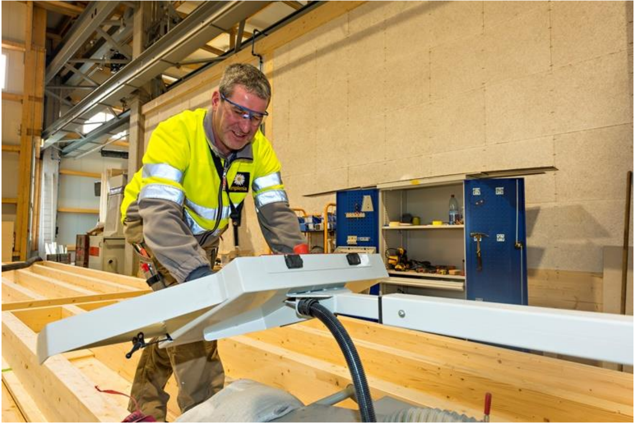
Implenia is investing in wood construction: the new production hall in Rümlang uses end-to-end digitalised processes. (Picture: Implenia)
