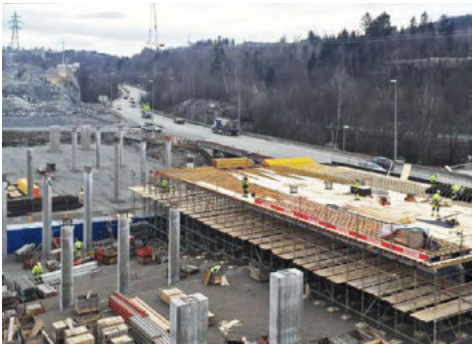
The old bridge piers on the E16 Rud – Vøyenenga highway in Norway are not being thrown away but have been given away to a new user. The new bridge piers were built in March 2016.
