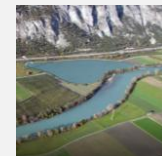
Imst-Haiming Hydrop. Plant
