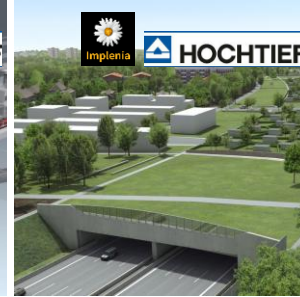
Hamburg-Altona Tunnel A7, DE
