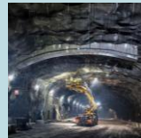
Johannelund bypass, Stockholm, Sweden
