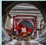
2 nd Gotthard Road tunnel, Switzerland
