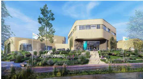
BCL (construction site logistics): Rebstockbad, Frankfurt, Germany
