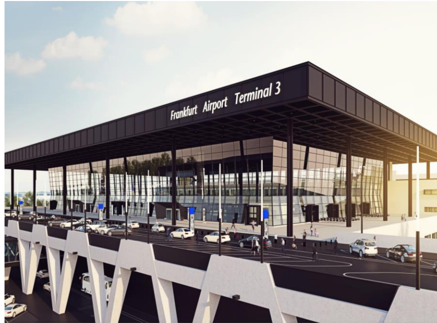
Facade technology: Airport Terminal 3, Frankfurt, Germany
