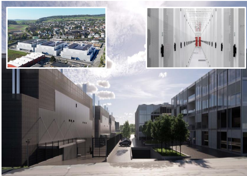
Data centre Metro-Campus, Zurich, Switzerland
