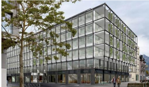
Children’s/women’s clinic, Lucerne Cantonal Hospital, Switzerland
