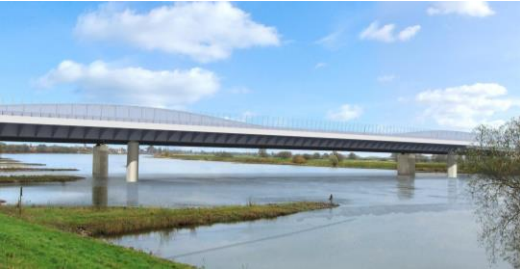
BBV Systems (post-tensioning): Elbbrücke Wittenberge, Germany
