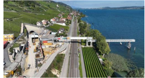
Ligerz Tunnel, CH
