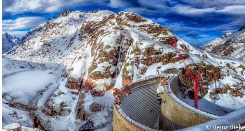
Spitallamm dam, Grimsel, CH
