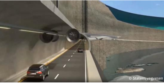
Rogfast Tunnel, Kvitsøy, Norwegen
