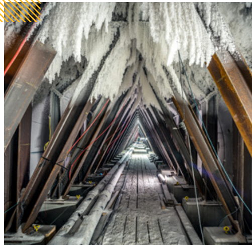
The biggest city-centre ground-freezing in Europe, right in the middle of Berlin and 20 m below the Spree Canal
