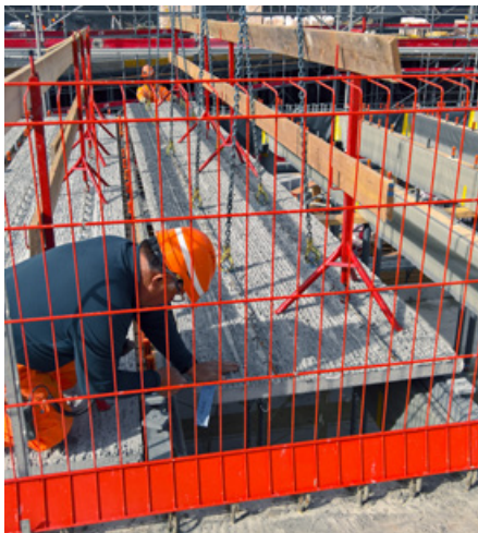
Pre-mounted fall protection These pre-mounted railings mean suspended ceilings can be installed more safely.
